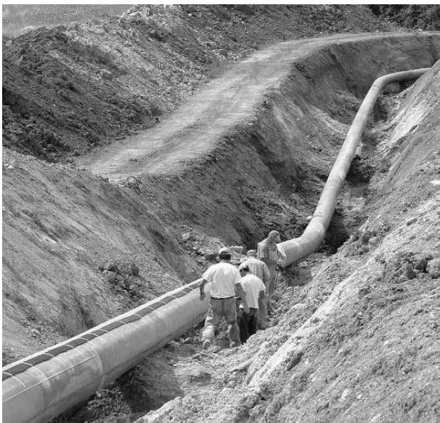
Fig. 19: SMARTape on the gas pipeline.
