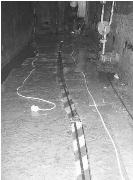
Fig. 18: SMARTape installation in the inspection gallery
