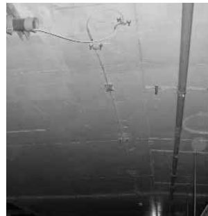
Long-gauge SOFO fiber optic sensor
